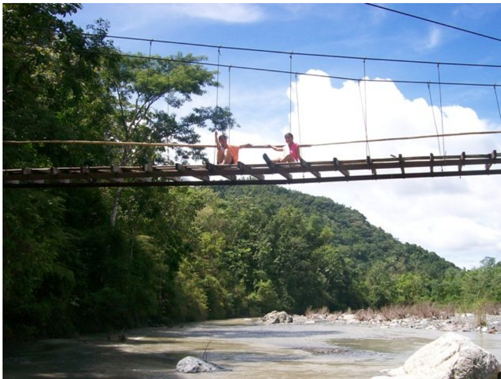
Figure 11. Hanging bridge constructed inside the park
