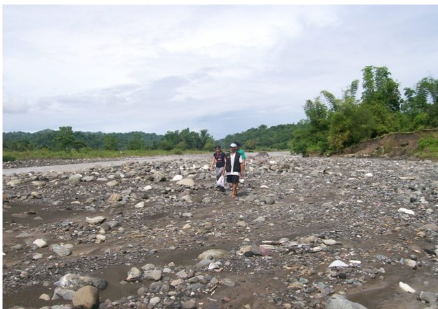
b. Eroded river bank inside the park
