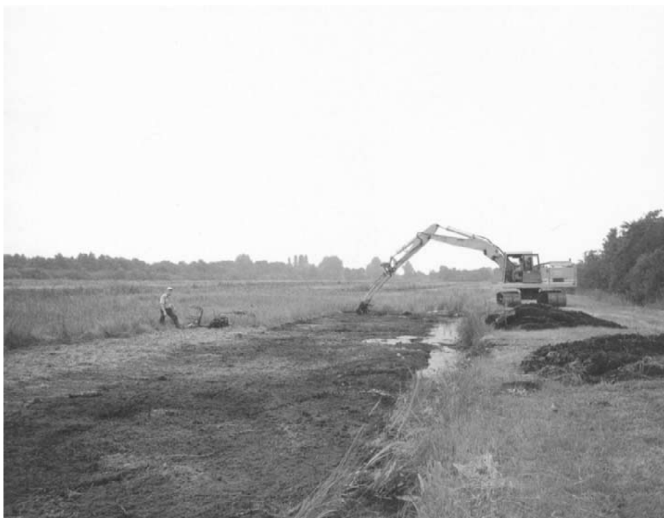
Figure 7. Restoration of quagfen vegetation by the mechanical removal of the top layer. In this way, succession is reset. Photo: B. Beltman.
